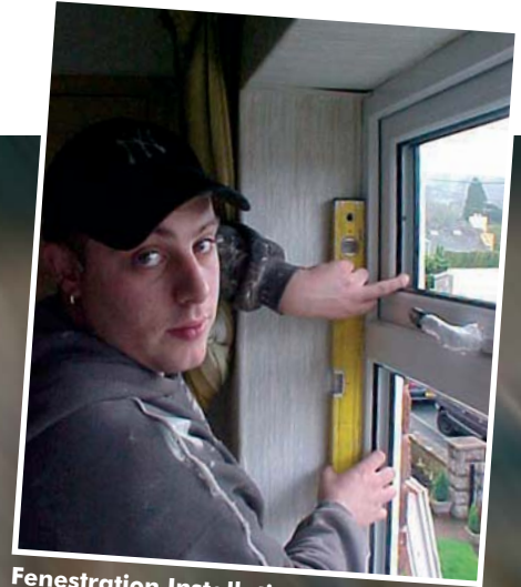
Fenestration Installation Level 2 Nicky John Miller of MNA Installation via Advisory Management Services
